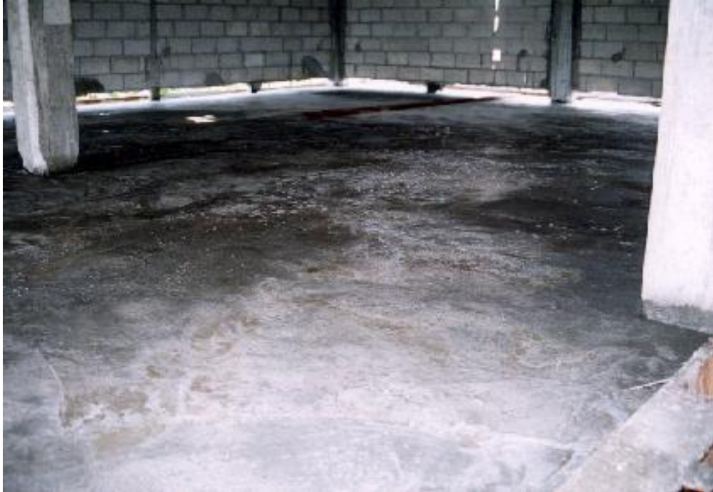
1/3 of the second floor poured
