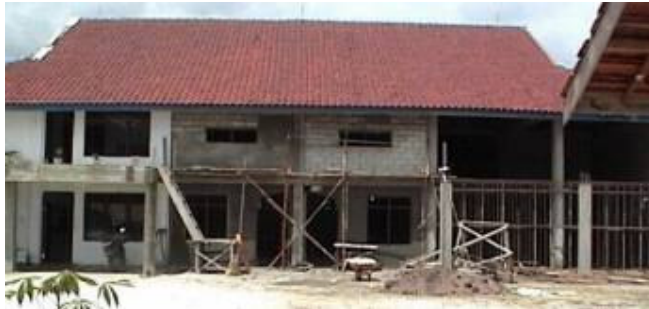
in the centre of the building
