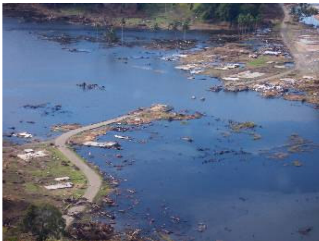
One of many bridges destroyed and much of the road system along the coast
